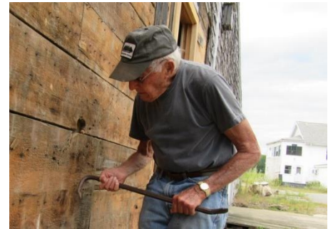
Mill volunteer, Bob Kline, pulls nails to prepare for re-shingling on the wall facing Rt. 130.
